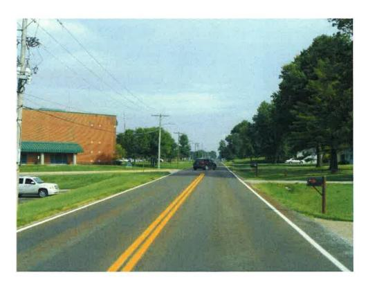
Photo 5: Southern high school entrance, just north of 155<sup>th</sup> Street and Parallel Road intersection, looking north. No turn lanes into high school, causing stacking.
